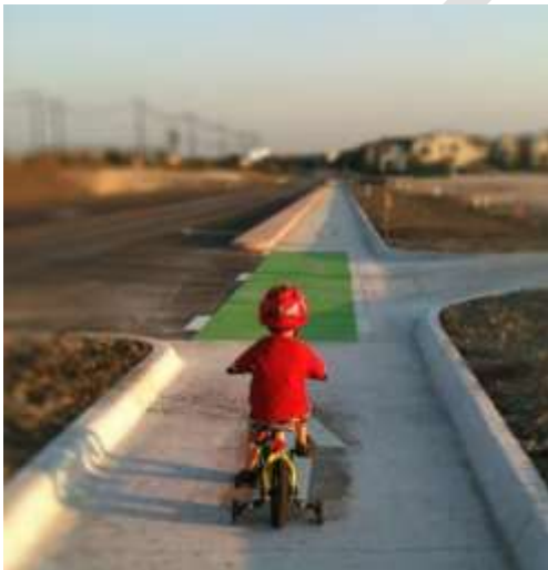
Caption: New protected bicycle lanes on Berkman Drive as part of the Mueller Redevelopment project (Photo courtesy of Greg Griffin).
