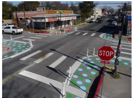
ATD engineers redesigned this pedestrian-rich, crash-prone intersection at E. 6th and Waller to make it safer – especially for people walking.
