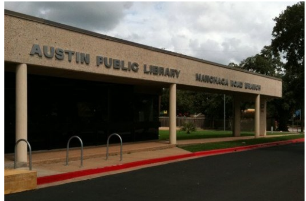
Austin Public Libraries are cornerstones of public access to technology in our communities. Manchaca Road Branch Library has computers available for use by local residents.
