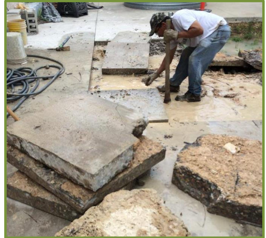
Parents of students at Perez volunteer to do some of the heavy lifting as they begin installation of the Courtyard Pond.
