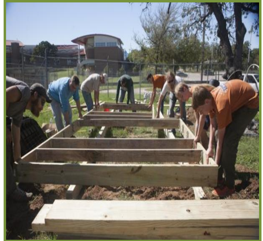
Kealing students and volunteers build the tool shed that will be the centerpiece of the rain collection system.
