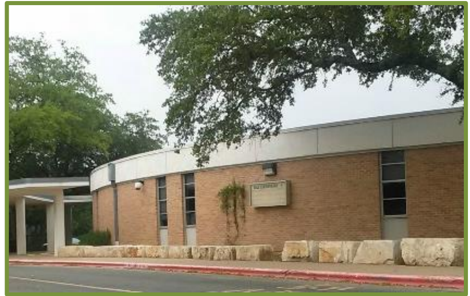
With over 70,000 square feet of flat roof space, Hill Elementary's rain collection system should capture enough water to provide campus irrigation.
