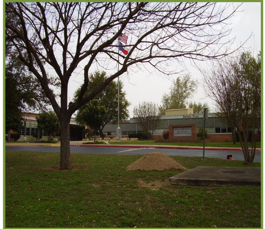
Preparations have begun for Travis High School's Outdoor Learning Center.
