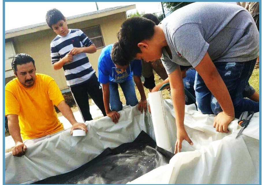
Parents and students helped construct garden beds that are watered from rain cisterns.
