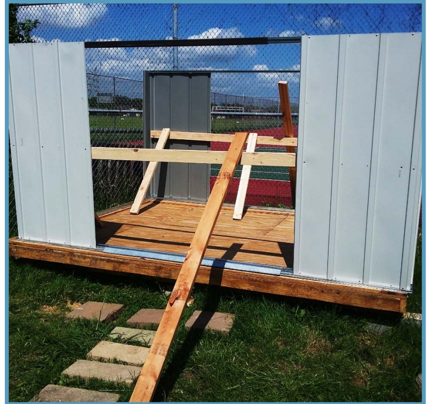
With this shed built out of repurposed materials, Covington students now have a secure place to store their gardening equipment..
