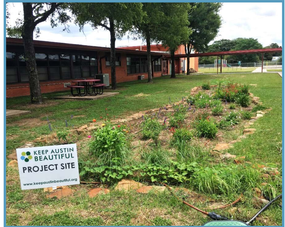
One of several garden beds at Sims that help with rain water run-off.
