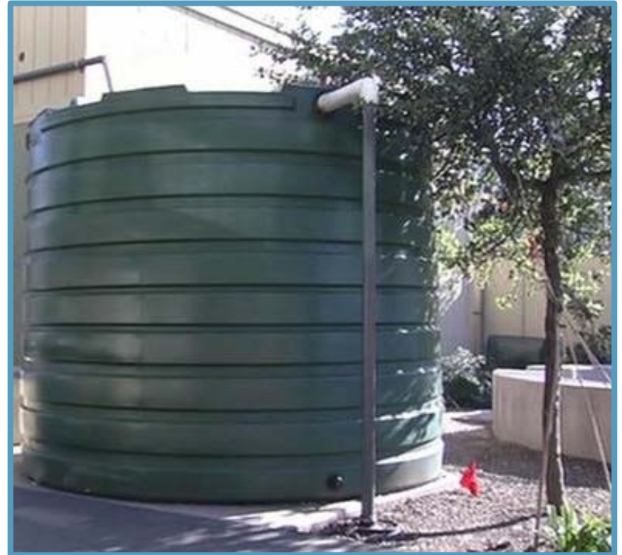
Rainwater collected in this cistern at Metz will provide water for campus landscaping.
