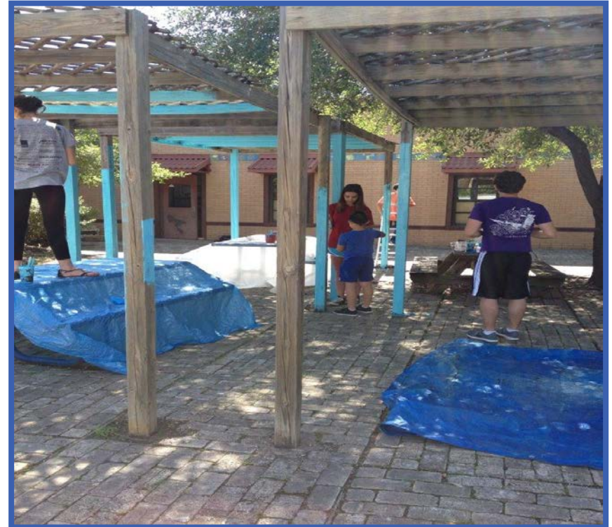
Metz Elementary School students helped construct their outdoor classroom.
