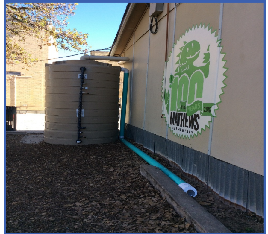
Rainwater collected from the roof will water garden beds at Mathews Elementary School.
