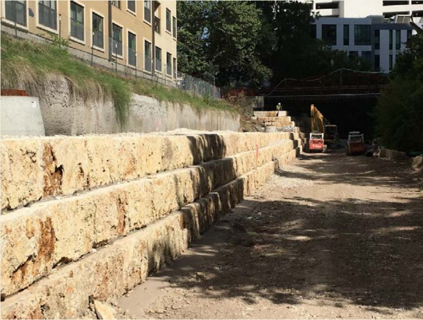
Shoal Creek, Bank Stabilization
