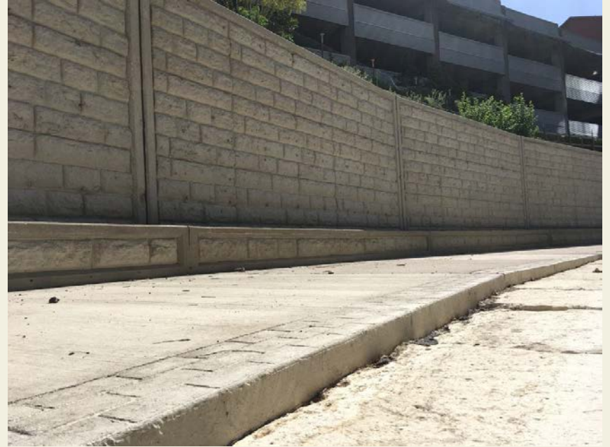
Shoal Creek Trail and Retaining Wall
