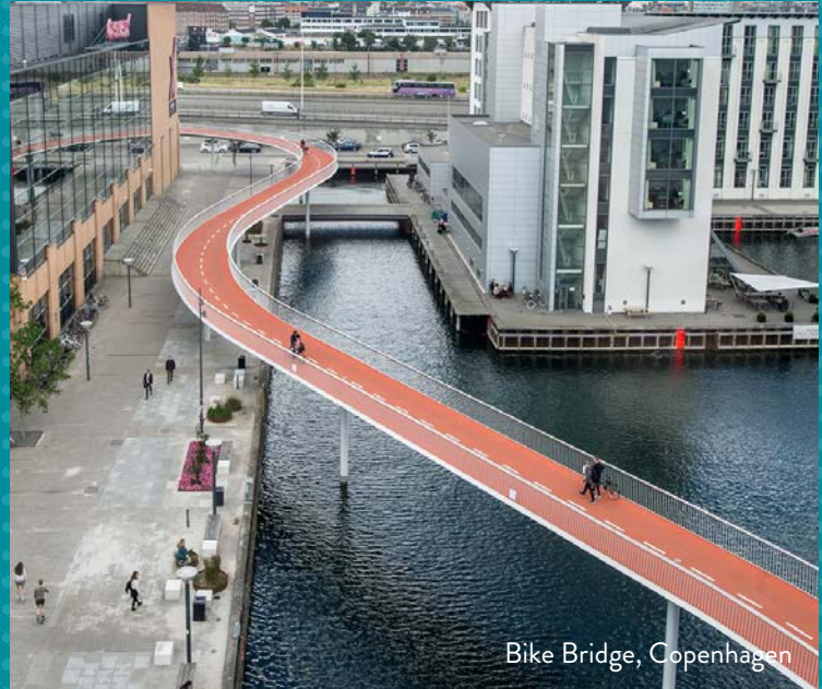
Bicycle or pedestrian bridge
