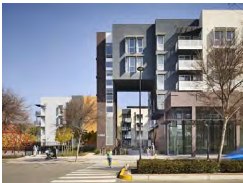
Station Center, Union City, CA
