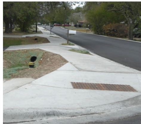
New sidewalks and improved drainage along Plains Trail—provides a safer route to McBee Elementary
