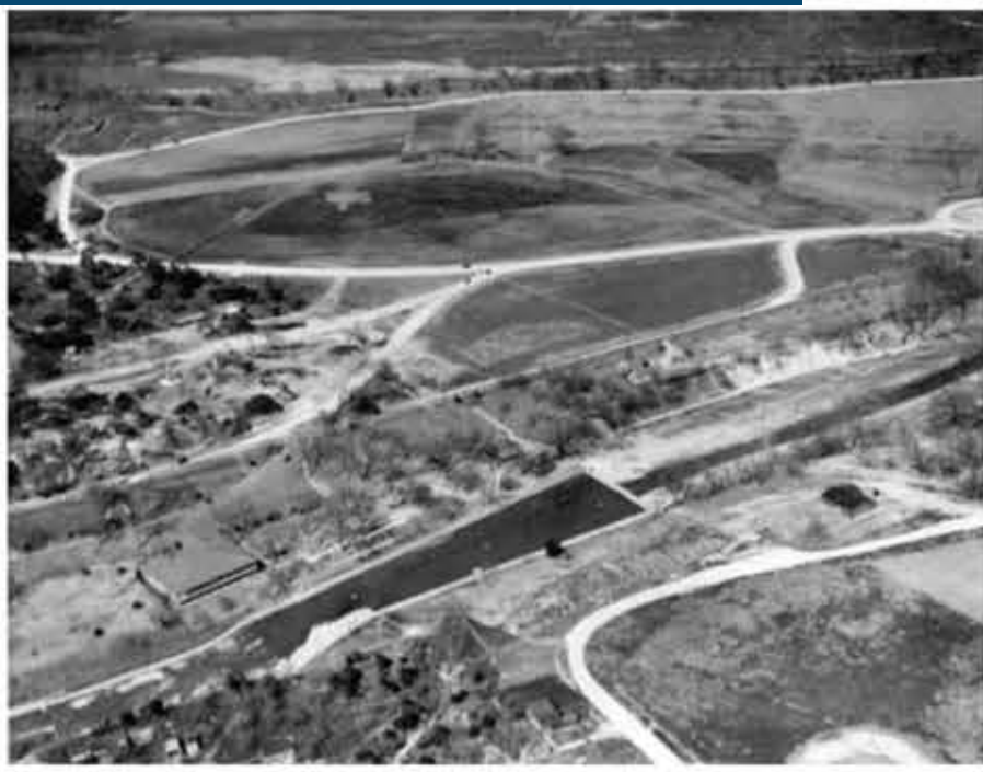
Aerial Photograph of Zilker Park (1935) Source: Austin History Center
