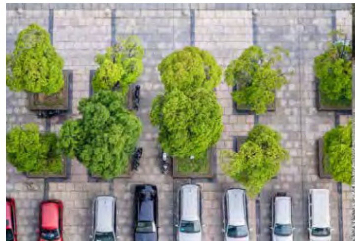
Permeable pavers (Image credit: Sherwood Design Engineers)
