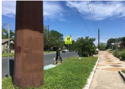
4. Electric transmission line
