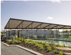
Concrete Walls & Steel Frame 5 votes
