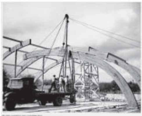
Doris Miller Auditorium under construction
