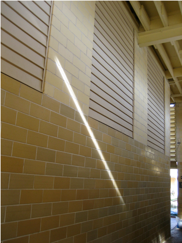
What were originally designed as generous openings into the basket rooms are covered with vinyl siding. A rehabilitated Bathhouse should replace the siding with glass to create a light-filled, double-height space.
