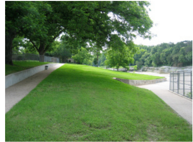
The slopes on the northside accessible route should be measured to verify that they meet the requirements of the ADA.
