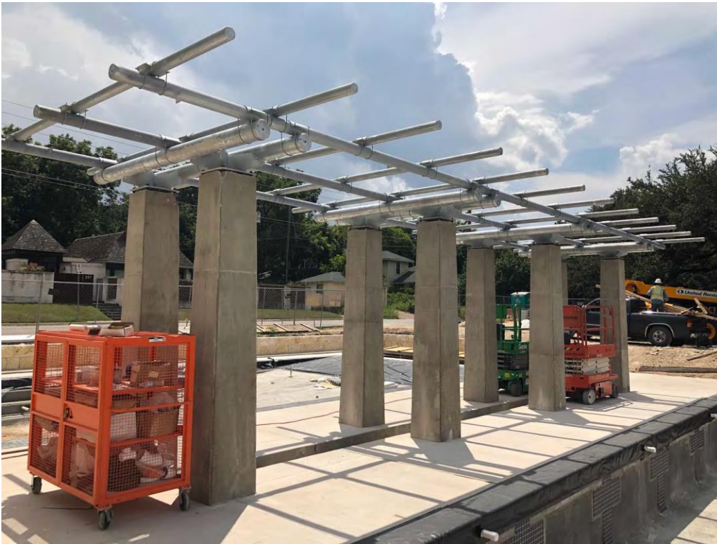
View of main shade structure
