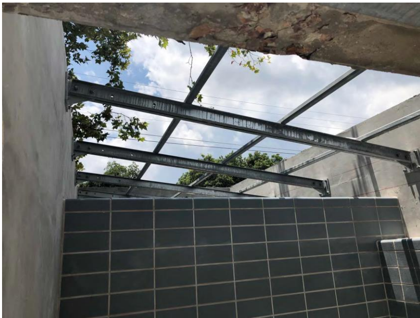
Interior view of glazed tile and roof support feature
