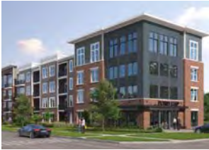
FLATS AT POND GAP Knoxville, TN
