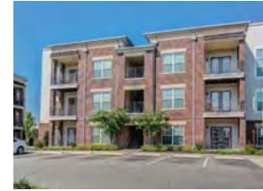
CRESCENT BLUFF I Memphis, TN
