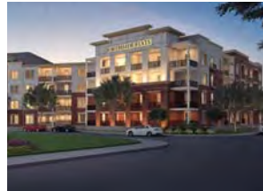
SOUTHSIDE FLATS Knoxville, TN
