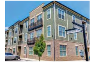
CRESCENT BLUFF II Memphis, TN
