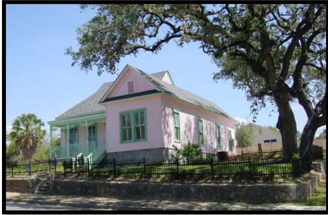
Connolly-Yerwood House Historic Rehabilitation
