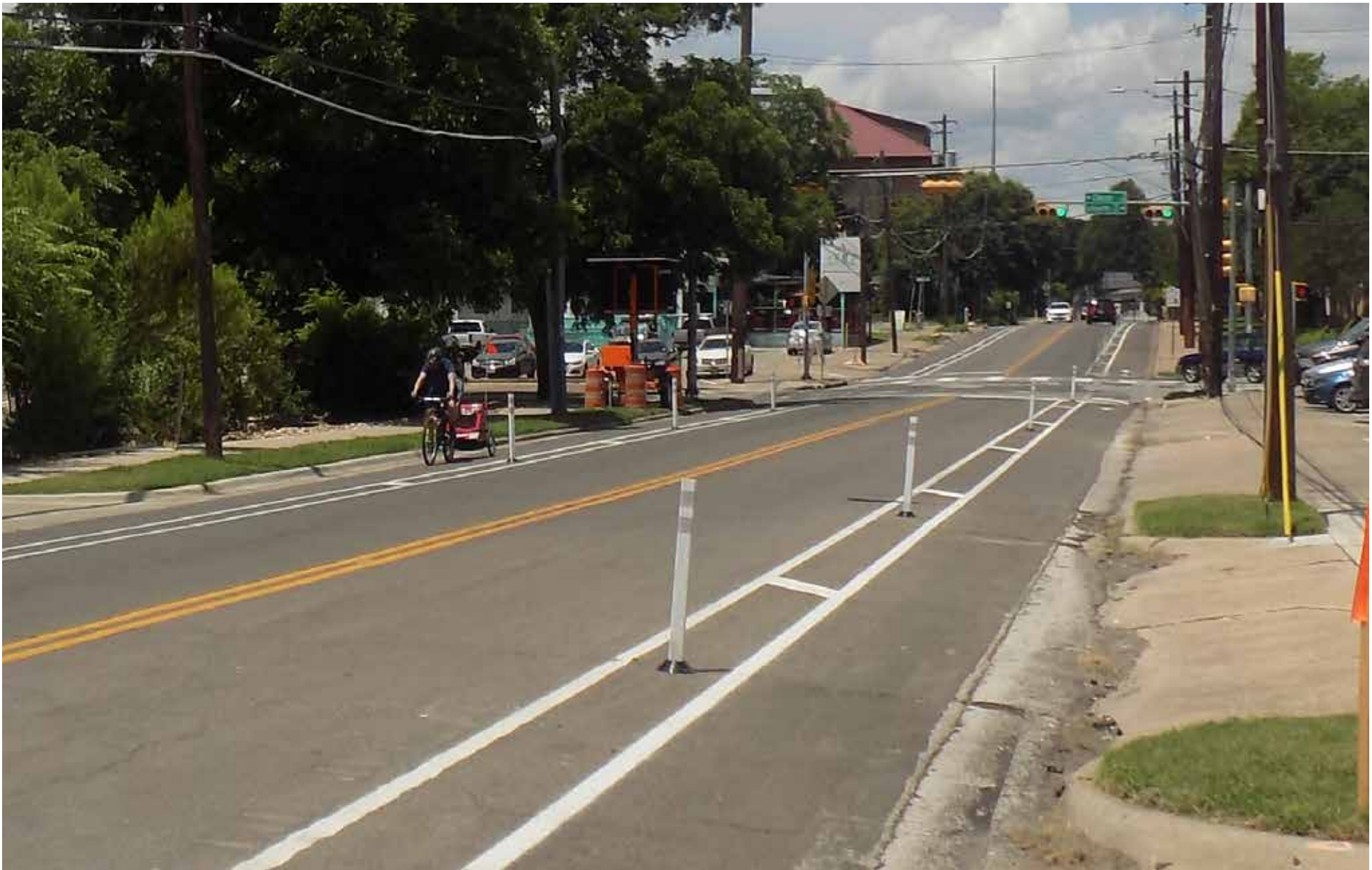
Example of one-way protected bicycle lanes on Manor Road constructed using flexible posts.
