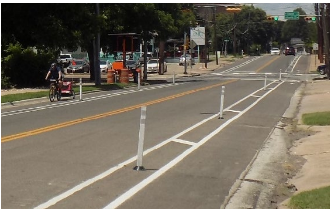
Examples of protected bicycle lanes and a pedestrian crossing islands constructed using flexible posts (“flex posts”) on Manor Road (left) and Berkman Drive (right)
