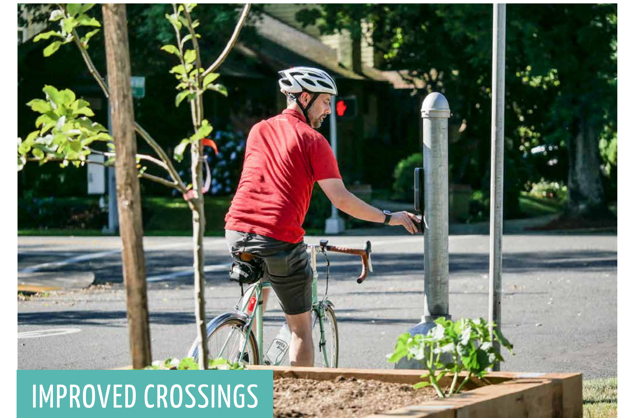
Placing push buttons close to the curb makes it easier for people bicycling to request to cross at a traffic signal on a busier street. Photo: Portland, Oregon
