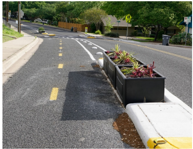
Example of pedestrian crossing islands and a two-way protected bikeway constructed using concrete traffic buttons and planters on Barton Hills Drive
