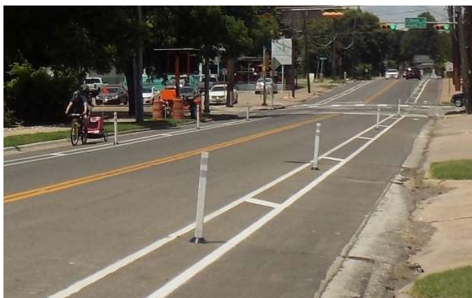
Examples of protected bicycle lane constructed using flexible posts (“flex posts”) on Manor Rd (left), and a pedestrian crossing island on Berkman Drive (right)
