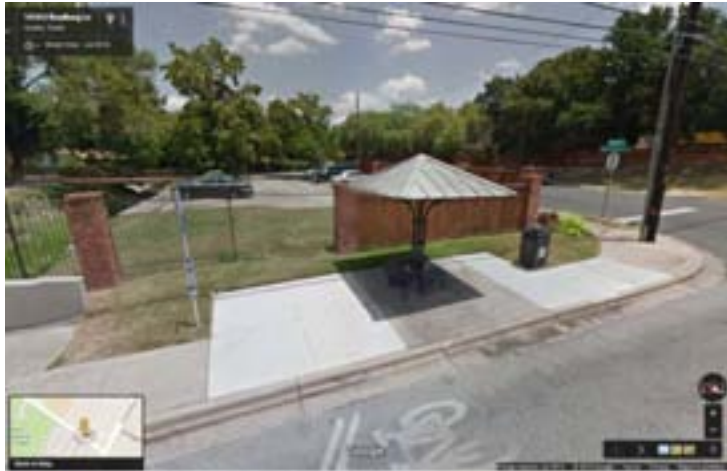
Stop #3125 Marlborough Drive and Rundberg Lane -North Side
