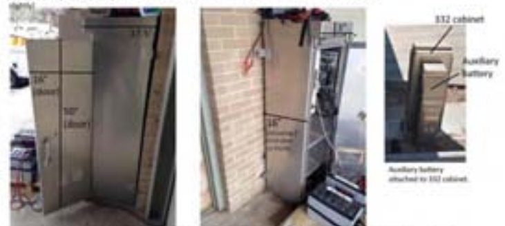
Auxiliary battery (attached to some 332 (tall) boxes - typically centered on the side but can vary)
