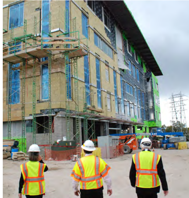
The New Central Library is currently under construction in the Seaholm Redevelopment District. Funded primarily by the 2006 Bond Program, the “Library of the Future” will be open to the public in late 2016.
