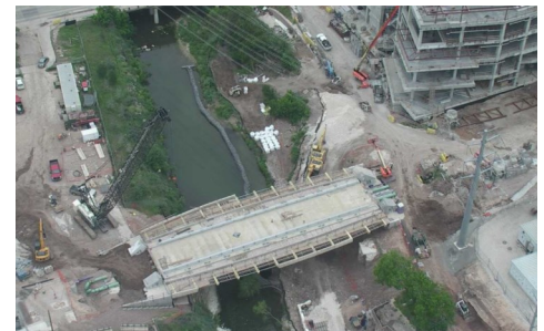
(Above) A recent photo of the construction of the New Central Library. (Below) A photo of construction of the Second Street Bridge.
