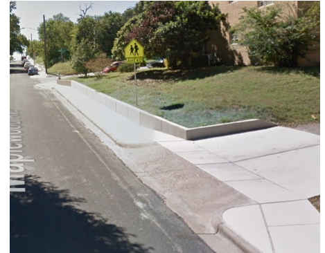
(Bottom left) Before picture of Maplewood Avenue near Maplewood Elementary School. (Below) After picture of Maplewood Avenue with new sidewalks and signage.
