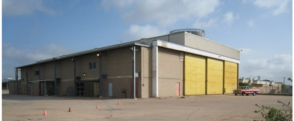
The 2012 Bond Program investment in Austin Studios will include renovations and improvements to the former National Guard Armory, pictured above.
