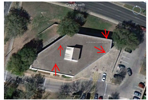
The roof of the Pleasant Hill Branch Library is in need of replacement.
