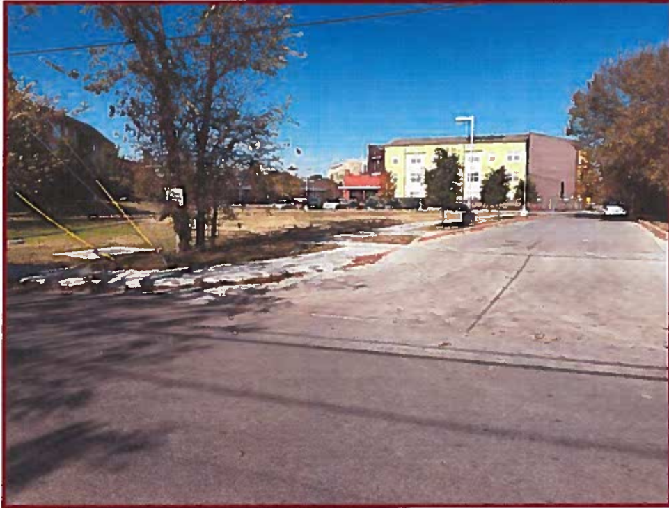
View of Subject Looking North
