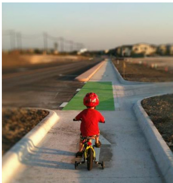
NEW PROTECTED BICYCLE LANES ON BERKMAN DRIVE AS PART OF THE MUELLER REDEVELOPMENT PROJECT
