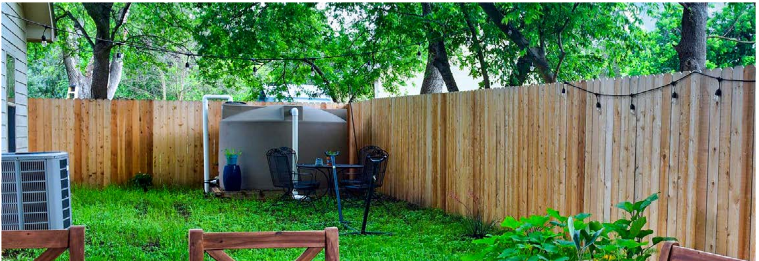
Figure 11d. Phase 2 Cistern installation
