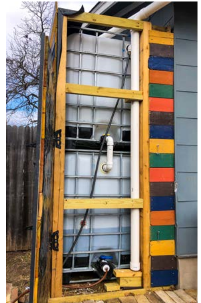
Figure 11c. Phase 2 DIY cistern installation
