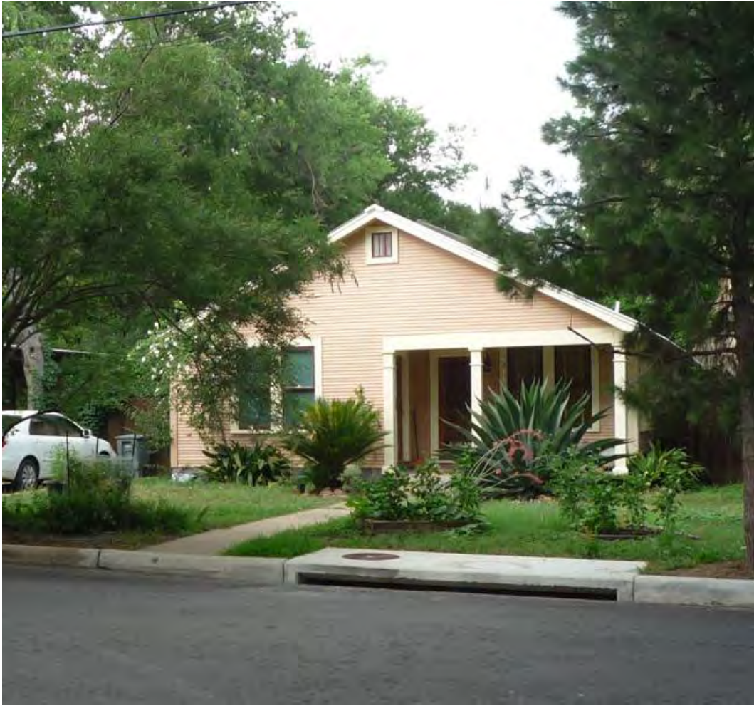
Storm Drain Inlets
