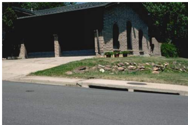
Photograph 7-4. Gutter/street slope is a major design factor for both street and inlet capacity.
