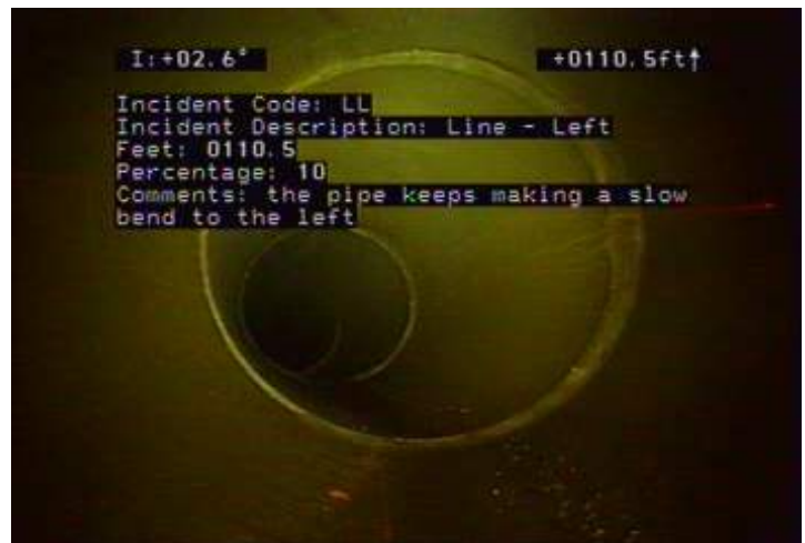
LL - Line - Left @ 110.5 ft. the pipe keeps making a slow bend to the left
