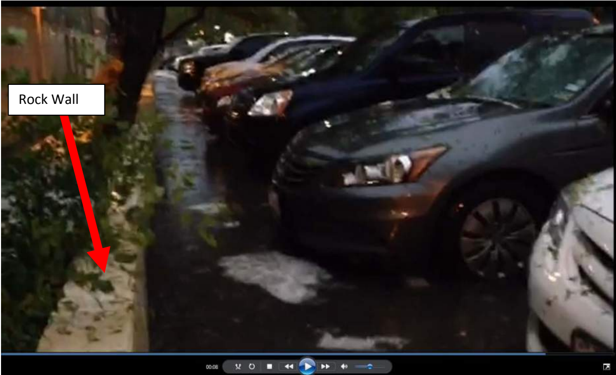
Photo 3 – rock wall constructed by Courtyard Condominiums to keep water out of complex
