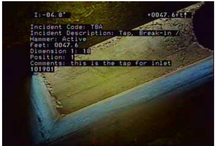
TBA - Tap, Break-in / Hammer: Active @ 47.6 ft. this is the tap for inlet 101901
