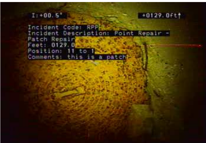
RPP - Point Repair - Patch Repair @ 129.0 ft. this is a patch
