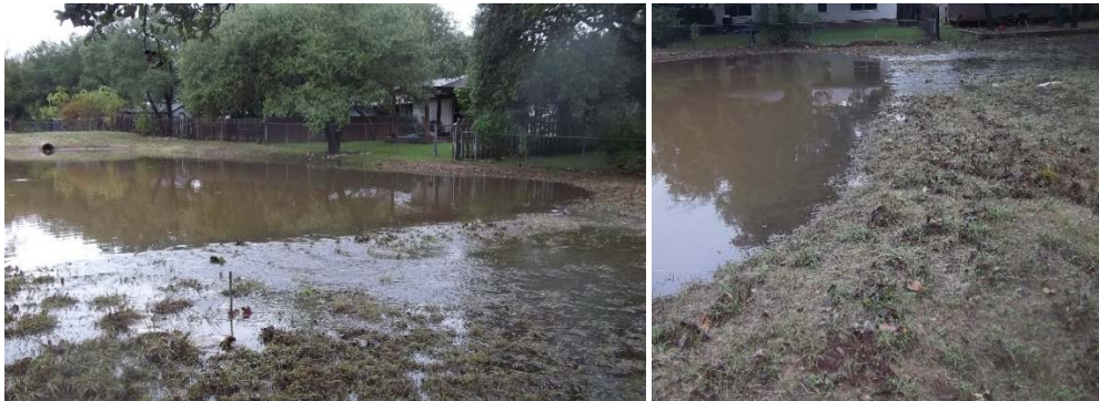
Nuisance flooding from the Maple Run Section 6 ponds
