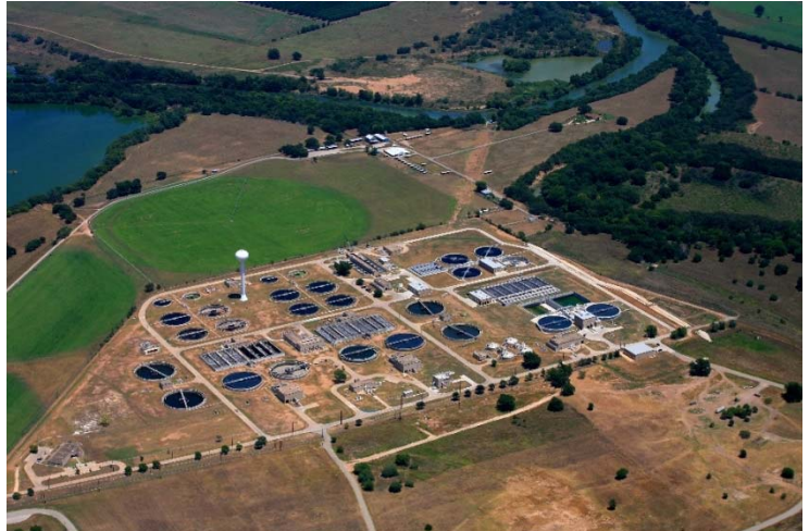
South Austin Regional Wastewater Treatment Plant (SAR WWTP)
