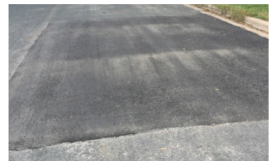
Street Cut Repair
