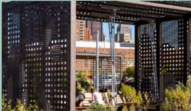
Perforated Metal Structure, Pier 26, New York
