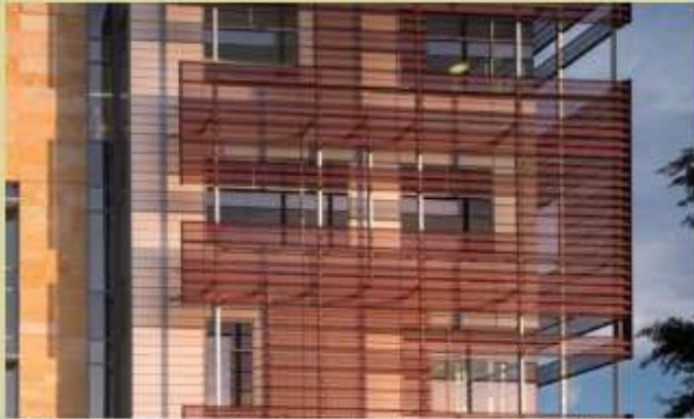
Perforated Metal Cladding, Austin Central Library
